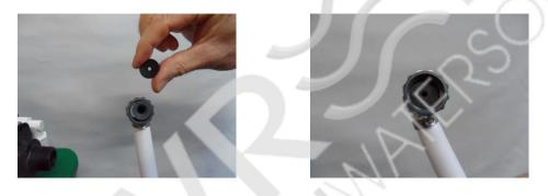
The Drain hose is then screwed onto the central drain port on the manifold, Hand tighten then just adjust slightly with grips to ensure water-tight fit. The direction of the drain hose can be fitted in any direction that best suits the installation position
